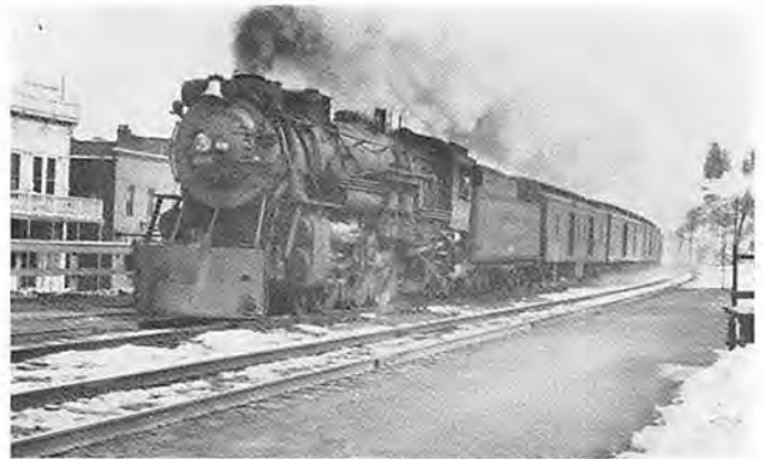
No passengers from the big city today. Pacific No. 6606, with the Scenic Limited in tow, speeds without pause through New Haven on a cold February day in 1939. In better weather, the balcony on the white fronted building to the left would have been a great place from which to watch this action. The date on its vertical cornice reads 1894. It is unchanged as of this writing.
